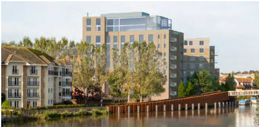
Figure 35 - Zoomed in extract of the summer view P6A from Reading Bridge, with Block D (foreground right), Block E (background far right) and the upper most floors of Block B (background left) – as existing (top), as approved (middle), as now proposed (bottom). Full versions are within Appendix 1.
